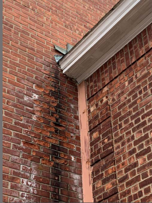
Slate roof repairs, soffit repairs, and masonry restoration at West Sand Lake
