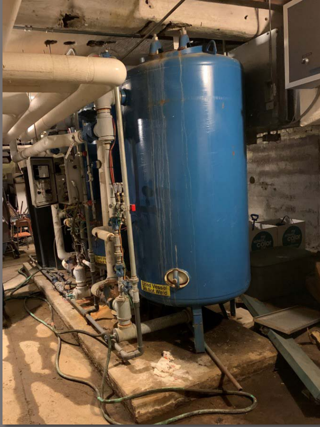
Boiler, water system, and circulating pump replacements at multiple buildings
