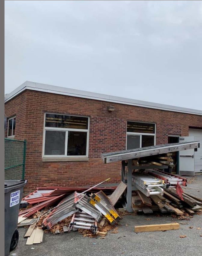
Area for Construction Technology Lab expansion
