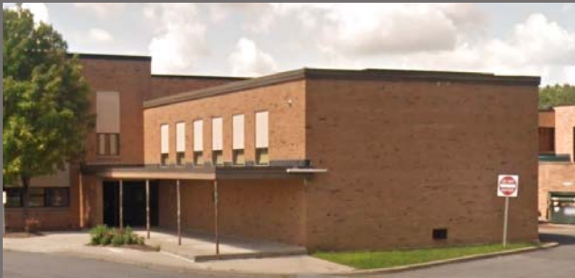
Existing cafeteria exterior
