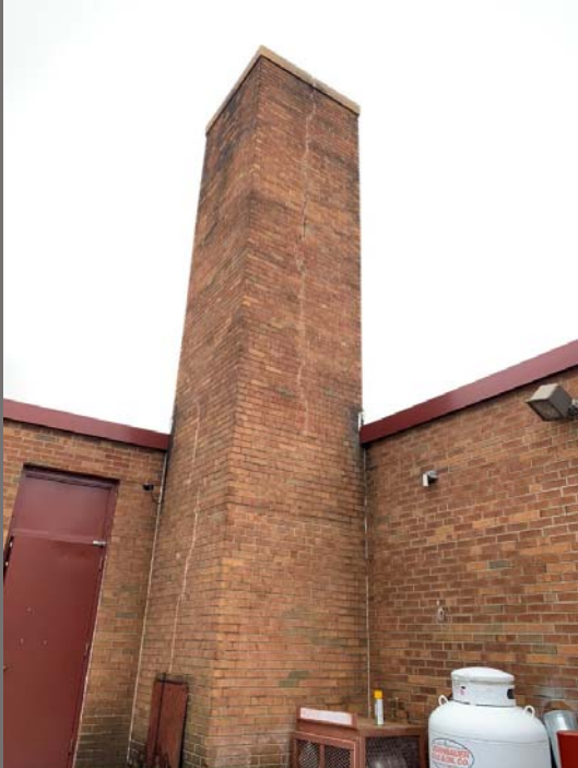
Chimney re-pointing and cap repairs at multiple buildings
