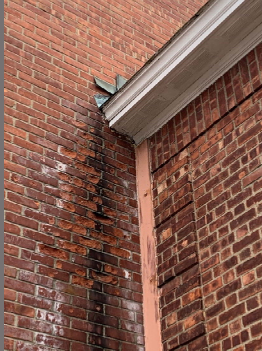
Slate roof repairs, soffit repairs, and masonry restoration at West Sand Lake
