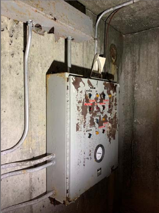
Electrical upgrades and various system replacements at multiple buildings
