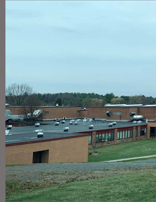
Roofing replacements at various buildings to address leaks, moisture issues, and warranties
